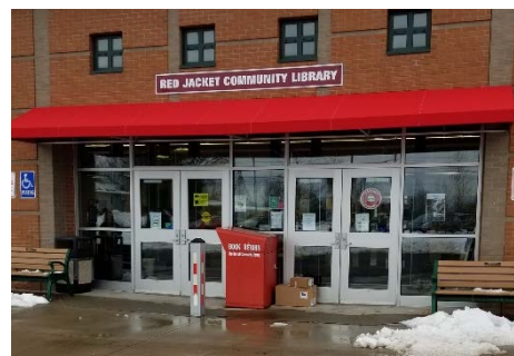
New sign and awning provided by the school
